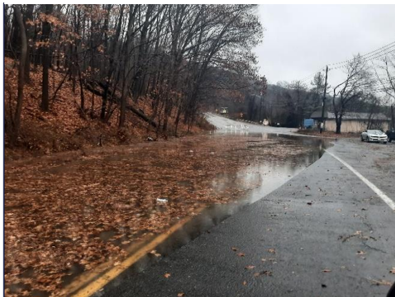
Figure 4.3.6-2. Stormwater/Urban Flooding in Rockland County
