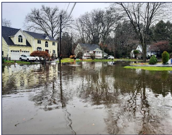
Figure 4.3.6-3. Stormwater/Urban Flooding in Rockland County
