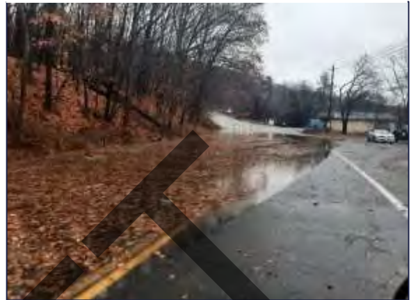
Figure 4.3.6-2. Stormwater/Urban Flooding in Rockland County
