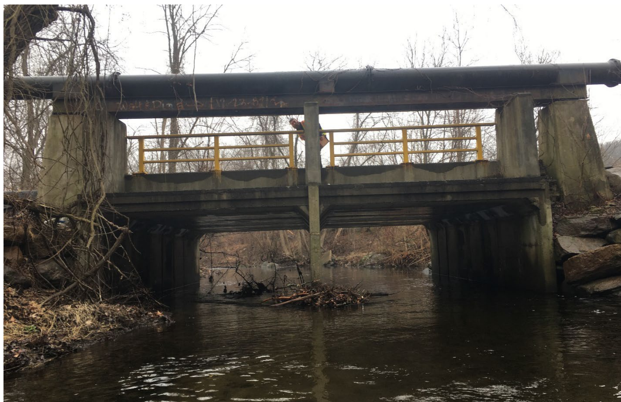
Figure 4-24: West Haverstraw DPW Facility Bridge
