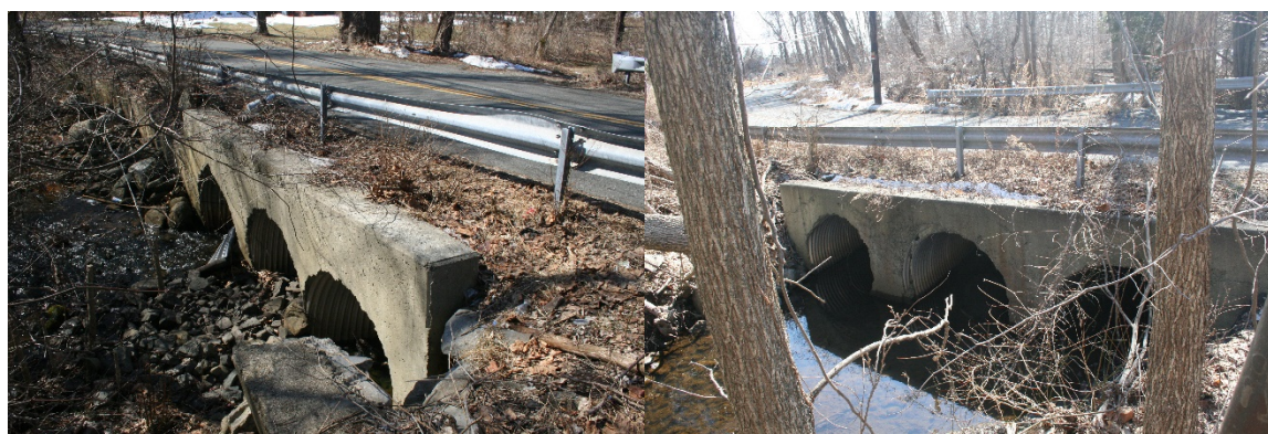
Figure 4-33: Inlet of Upstream Culverts (Left) and Outlet of Downstream Culverts (Right) on South Camphill Road
