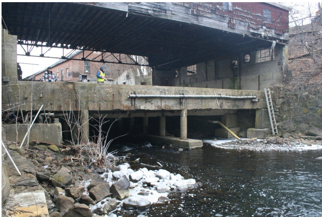
Figure 4-10: View looking downstream at Building 26A at the GAIC just downstream of the Bridge Street dam. Piers and other obstructions restrict flow and are prone to debris jamming.
