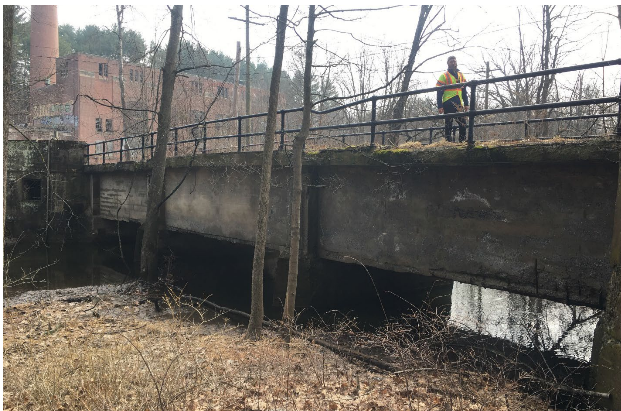
Figure 4-23: Rockland Print Company Power Plant Bridge
