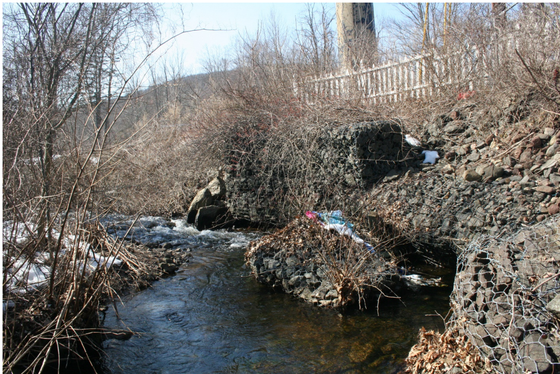
Figure 4-28: Gabions Falling into Minisceongo Creek Adjacent to Willow Grove Mobile Home Park
